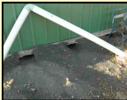
↑ Under concrete slabs.
