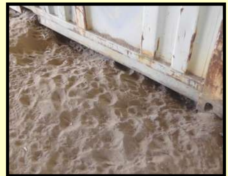
↑ Under shipping containers.
